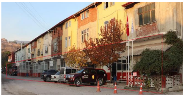
Figure 6. The Service Building of The Fire Department of Niksar Municipality
