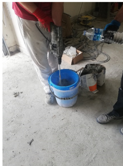
Preparation of repair mortar
