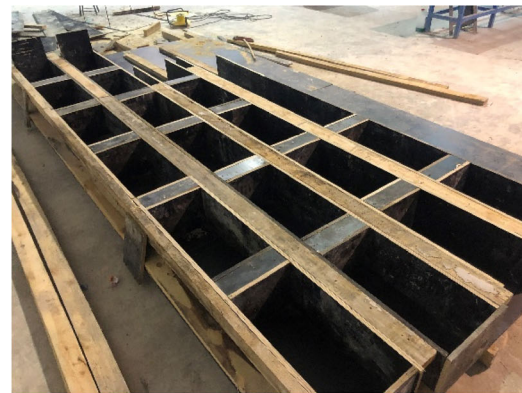
Completion of wooden formwork
