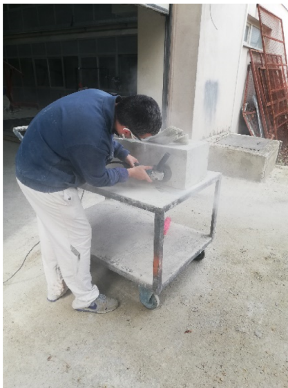
Grinding of concrete
