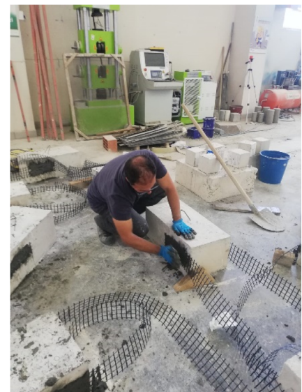
Bonding of TRM strip to the concrete surface
