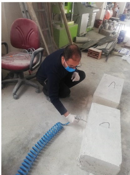
Removal of dust from the concrete surface
