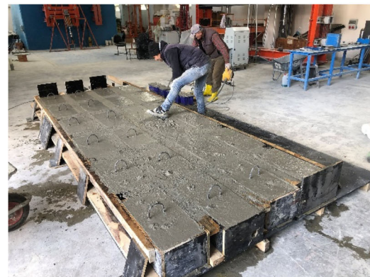
Placement of steel rings
