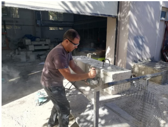
Grinding of the strip
