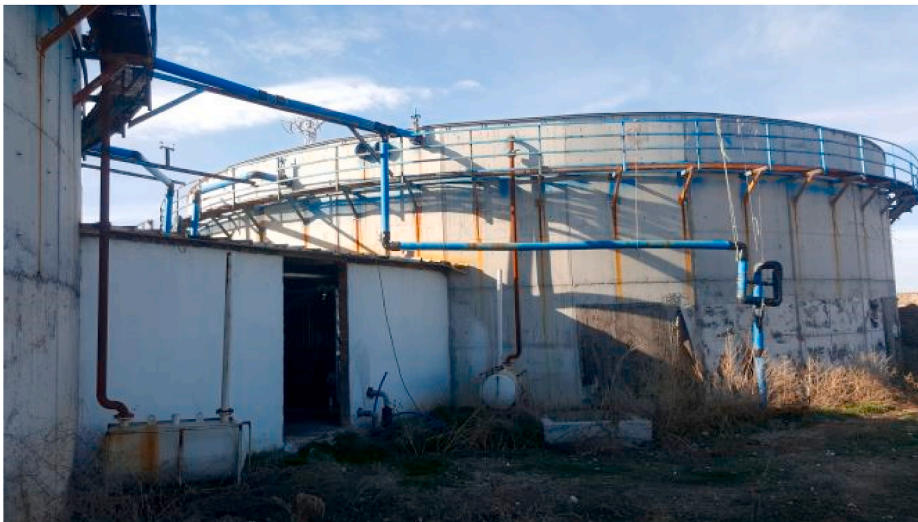
Fig. 2. The view of Pre-Digester, Post-Digester, and technical mechanical room.
