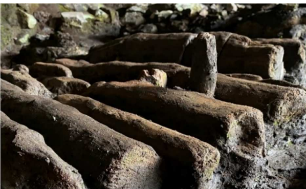
Figure 4. Piles driven between wooden bases.
