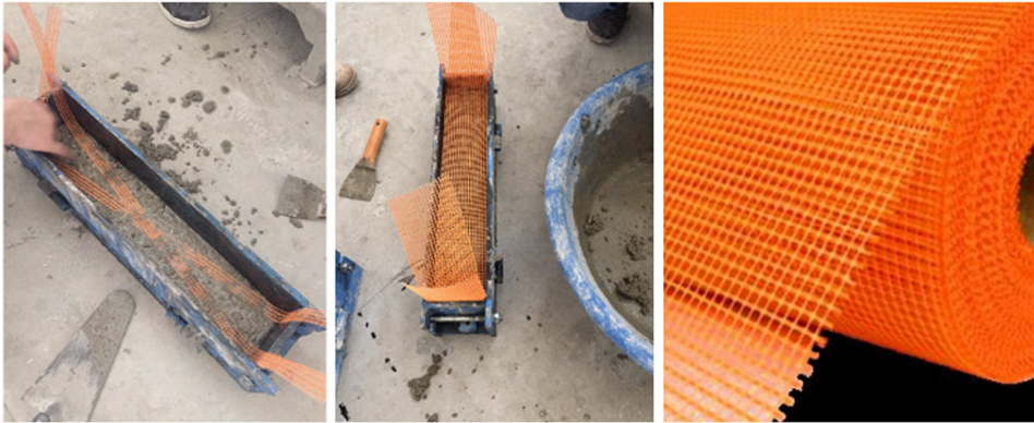
Figure 2: Placing GFM diagonally or straight into concrete beams.
