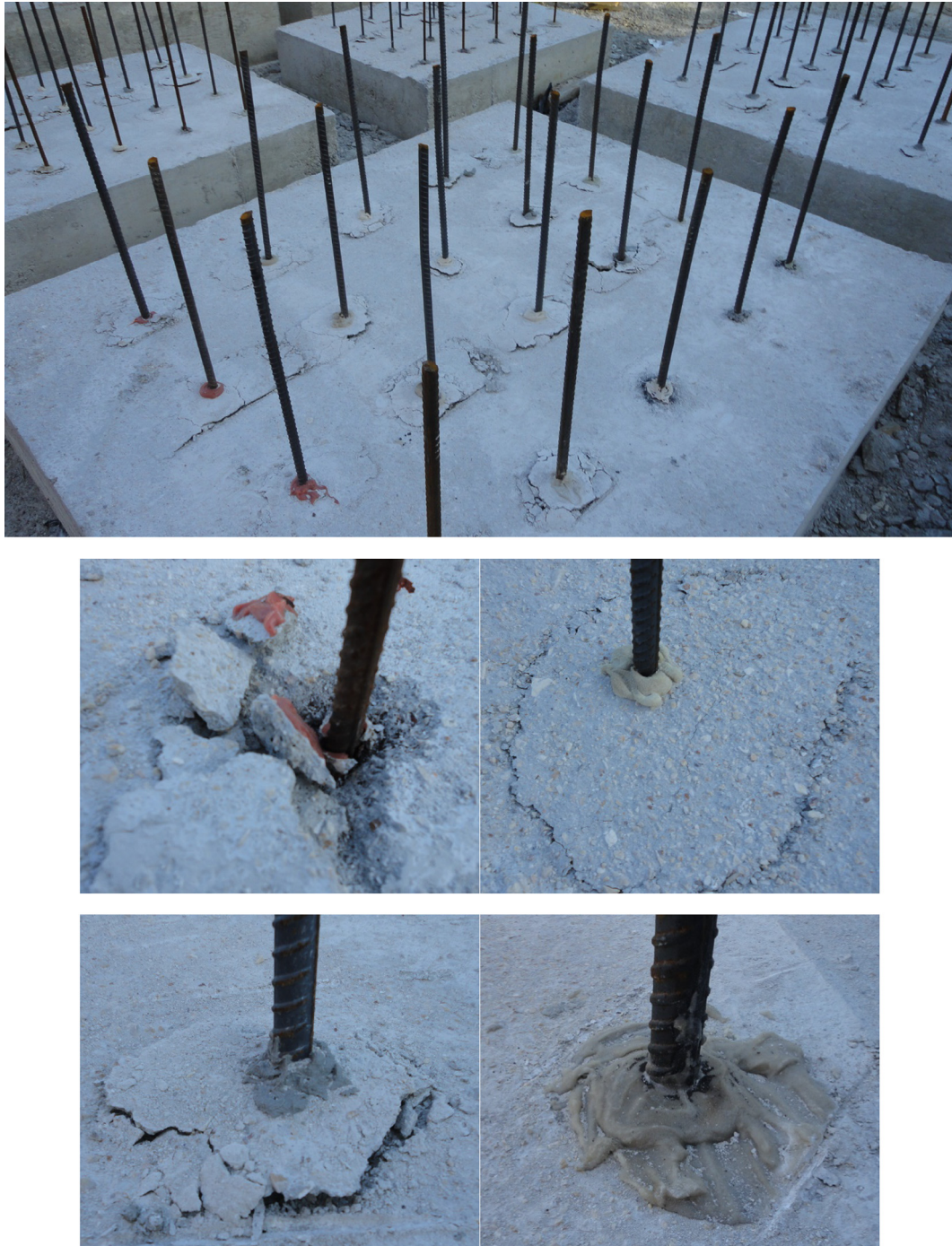
Fig. 5. Failure mechanism for some of the tested specimens.
