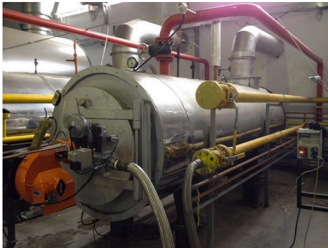
Fig. 1. ECO 45 G C 3B burner and boiler used for experimental study.
