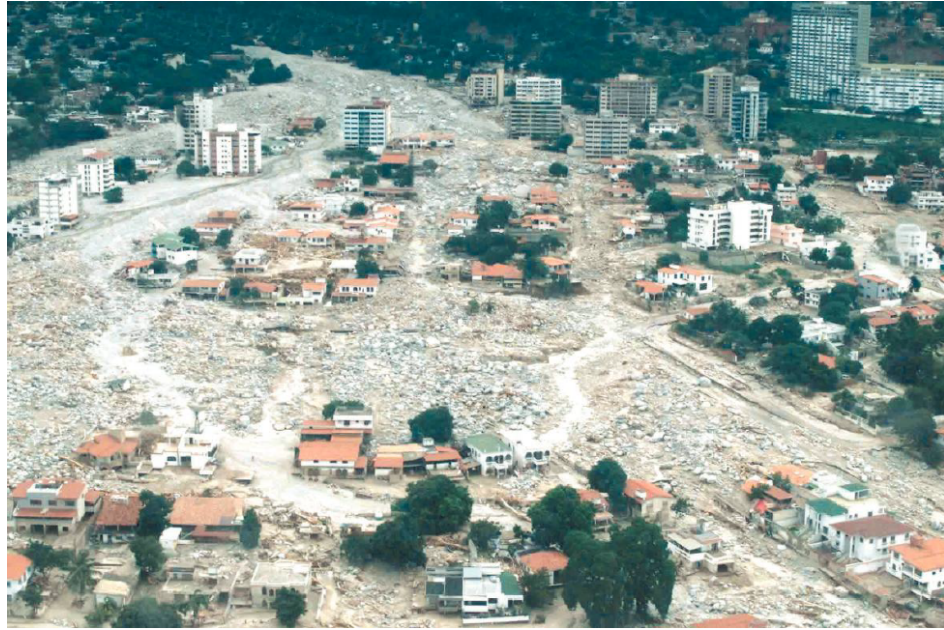
Şekil 3.6. Akma, Venezuela, 1999 (Fotograf: L.M.Smith, W.E.Station, US.Army Corps of Engineers) (Güler, 2017).
