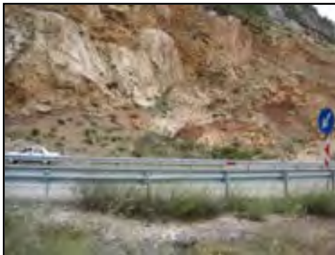
Figure5. The steep drop-off on the other side of the landslide
