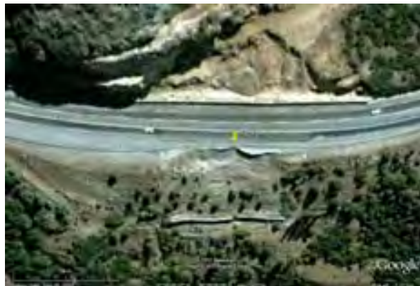
Figure 6.The satellite photo of the landslide in 2003.
