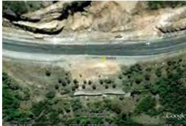
Figure 7. The satellite photo of the landslide in 2006.
